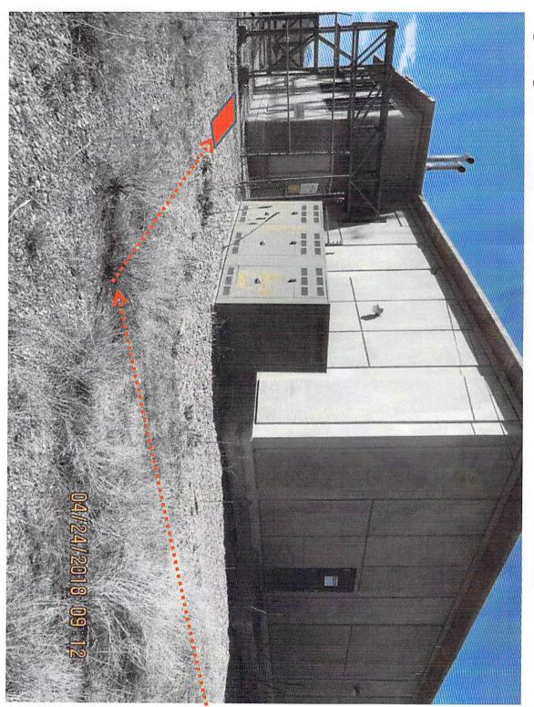
(N)17"x30" Hand Hole. (N)2" Conduit to be hand trenched through compound to the AT&T site.
